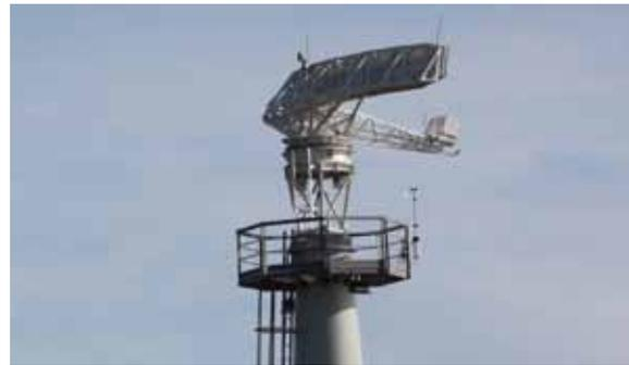
**Figure 3 - Coastal surveillance radar**
